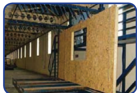
Frame UK Closed Panel Production
