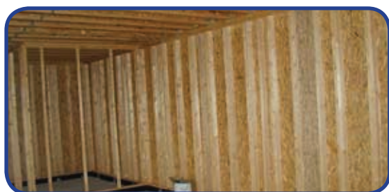
Open panel timber frame. Photo courtesy of Milner Associates (formerly CCB Evolution)
