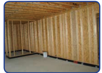
Open panel timber frame. Photo courtesy of Milner Associates (formerly CCB Evolution)
